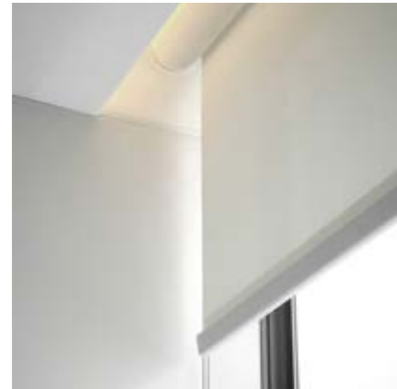
Indirect lighting in recessed ceilings
