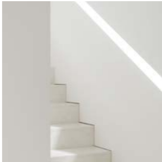
Indirect lighting in handrails
